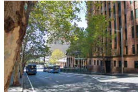
Phillip Street - existing
