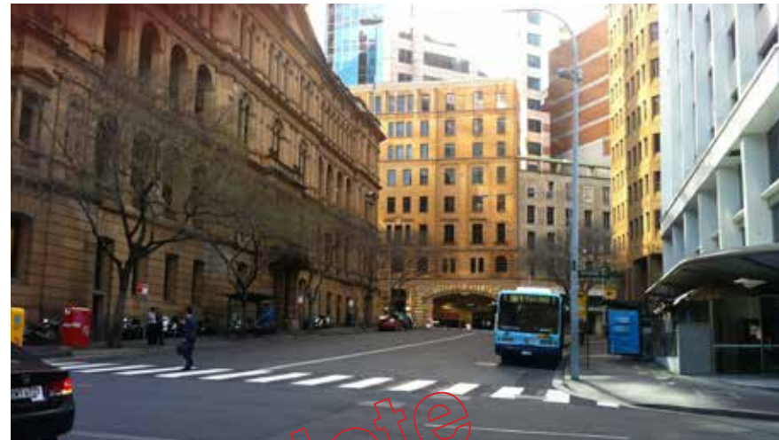
Gresham Street existing photo
