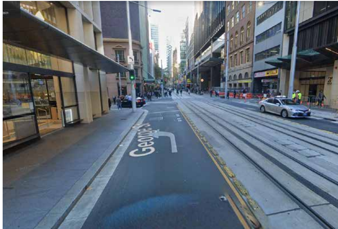
George Street north existing - view south towards Hunter Street showing narrow footpaths and high pedestrian volumes
